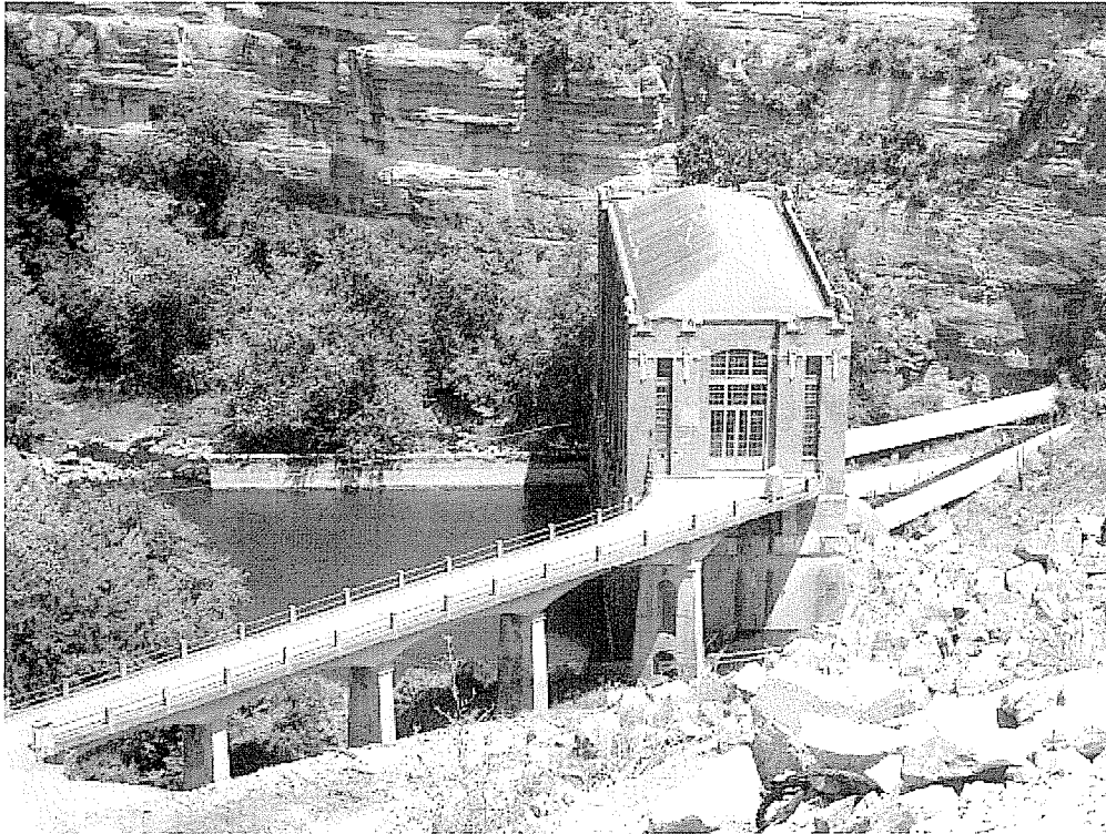
Figure 4.2-2 Dix Dam Generating Station
